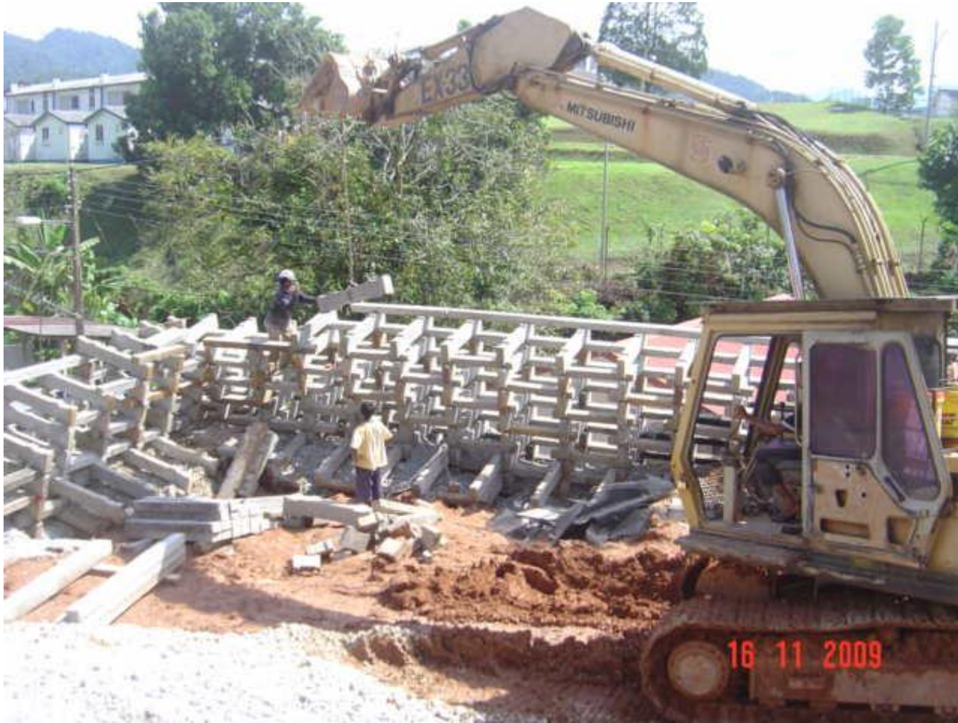
Concrete crib wall -
