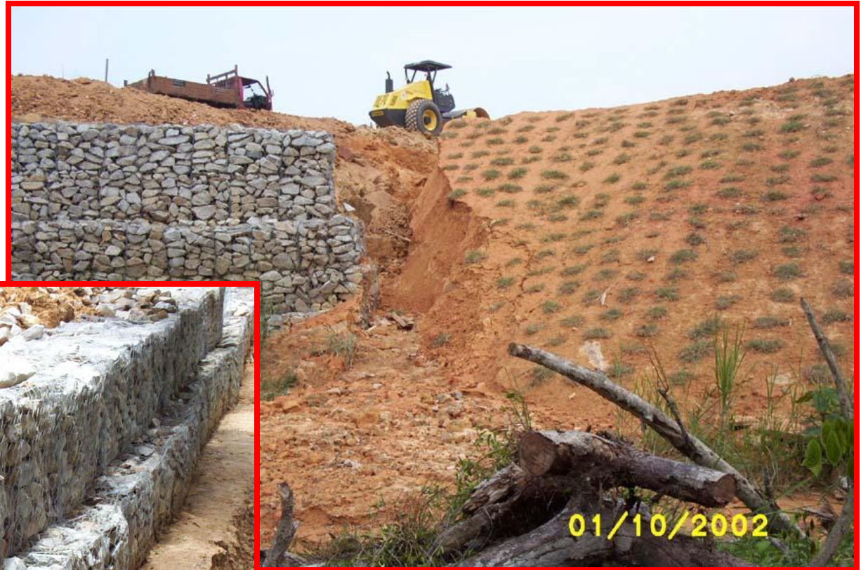
Spot Turfing & Gabion Wall
