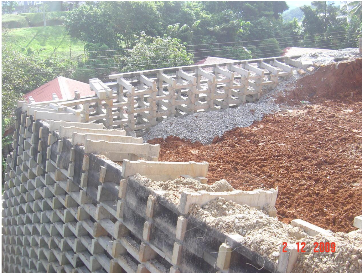
Concrete crib wall
