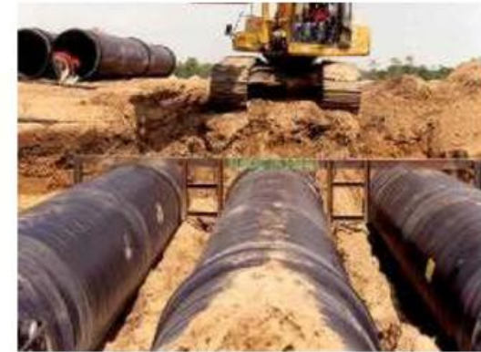
Storm water drainage system 60 in dia HDPE
